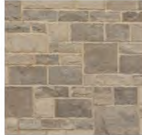
ST-1 STONE VENEER ECHELON MASONRY WATERFORD STONE "AVONDALE" (OR SIMILAR EQUAL) MORTAR COLOR: GIANT "SAND"
